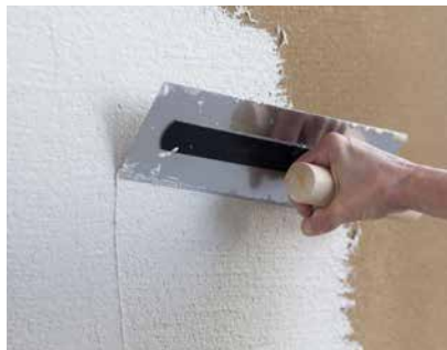
Apply mortar with the trowel.
