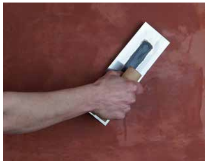
Stain filling execution
