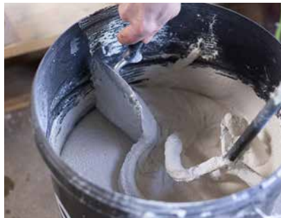
After 30 minutes, remix thoroughly. The image shows the ready-to-use consistency.
