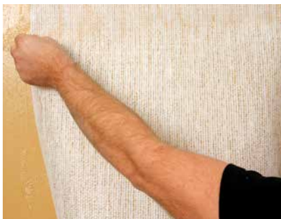
Pasting up glassfibre mesh wallpaper
