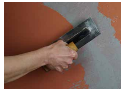
Applying the marbled topcoat
