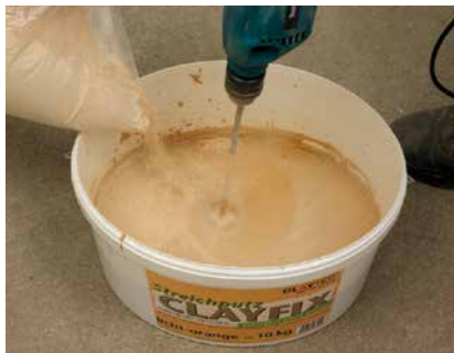
Mix bucket contents into water
