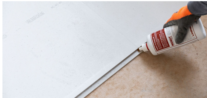
Photo: Laying the NORIT dry screed and bonding with the NORIT-TE adhesive
